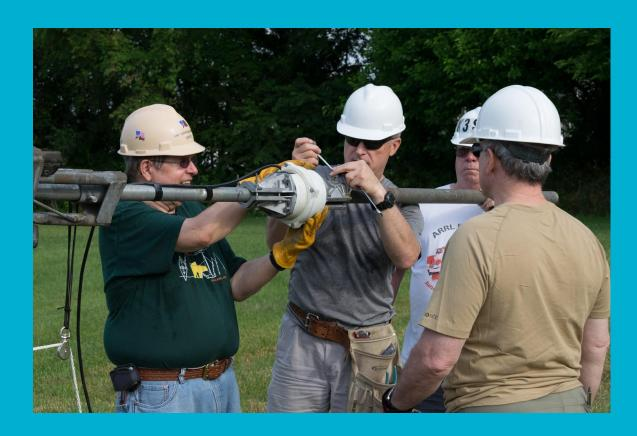
Attaching the antenna mast to the rotor
