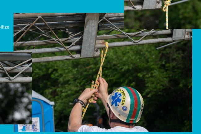
Attaching lines used to help stabilize the tower during raising
