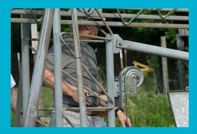
The side crank is used to change the angle of the tower to the ground
