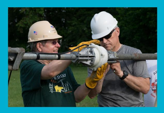
A pulley is attached near the top of the mast. The white rope pictured is used with the pulley to raise a wire antenna.
