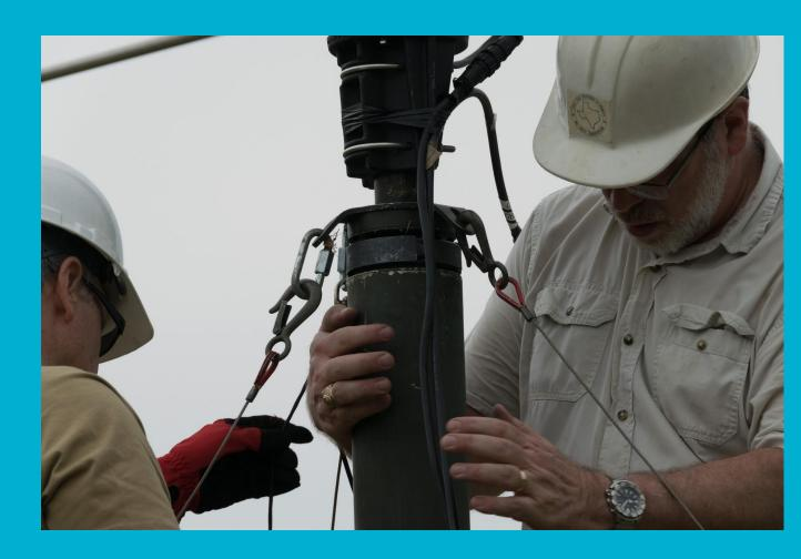
Unlocking the mast so it can be raised
